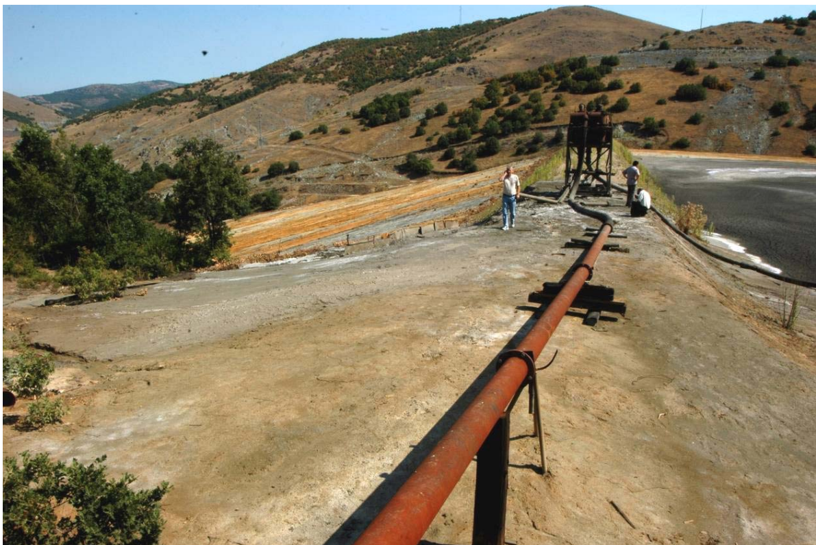
Photo 16 - Old tailings near the Badovac concentrator (site n° 2 of fig. 12), sampled by BRGM on the crest of the dam (sample n° 12 of Table 3); on the right, at the bottom of the dam can be seen the new tailings of sample n° 15 and photo 18
