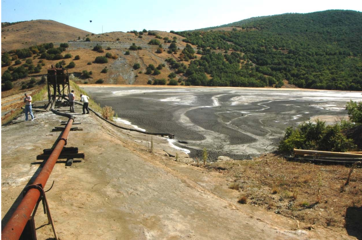
Photo 15 - Old (left side) and new tailings (right side) near the Badovac concentrator, sampled by BRGM (Site n° 2 of fig. 12)
