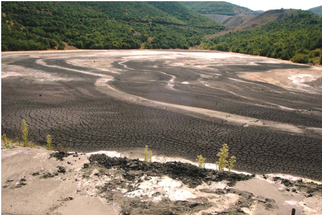
Photo 18 - New tailings (from the retreatment of the old tailings of the Marevc concentrator) near the Badovac concentrator (site n° 2 of fig. 12), sampled by BRGM down the crest of the dam (sample n° 15 of Table 3)
