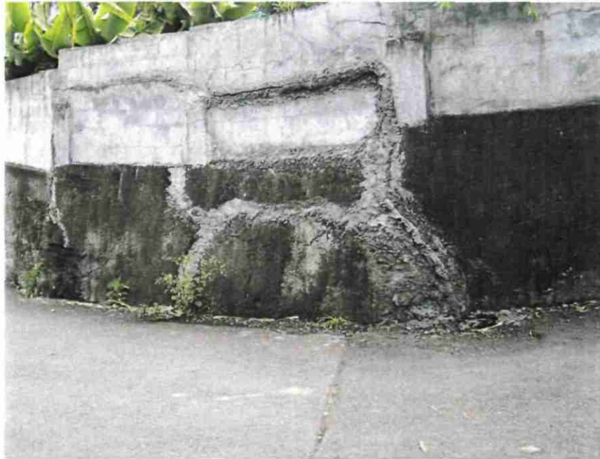
Figure 33 : Point 7 – Faille normale direction N140°
