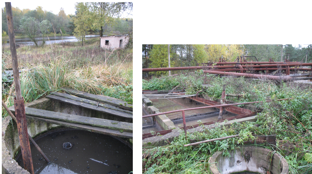
Figure 6. Unoperated waste water treatment plant in Gostitsy village.
