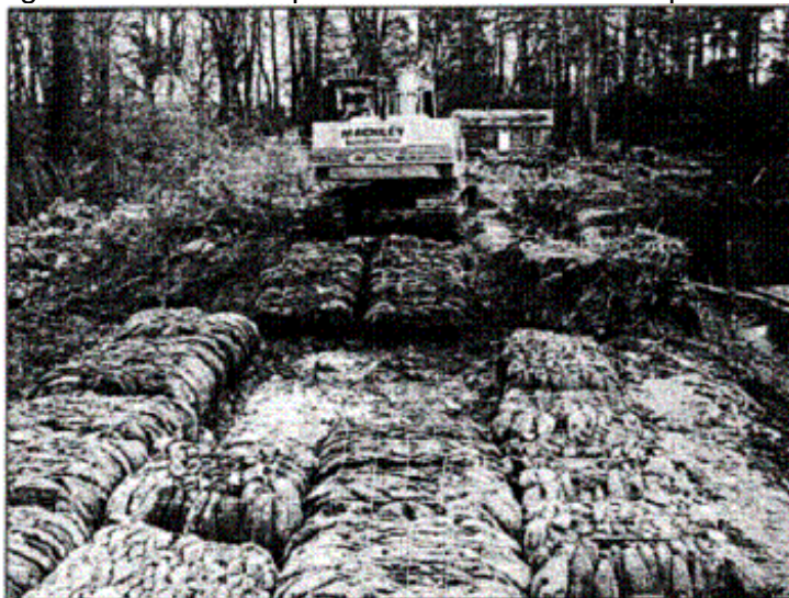
Tyres pressed into bales could be used for fill for walls and embankments.
